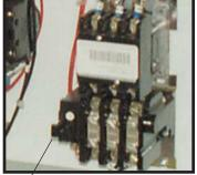
Reset level on overload relay
