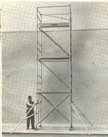
14 Adjustable Outriggers (above, left) or Long Adjustable Outriggers (above, right) may be used instead of outboard supports to provide the necessary base stability. Make sure each outrigger is wedged firmly against solid pavement and all clamps are tightened securely.
